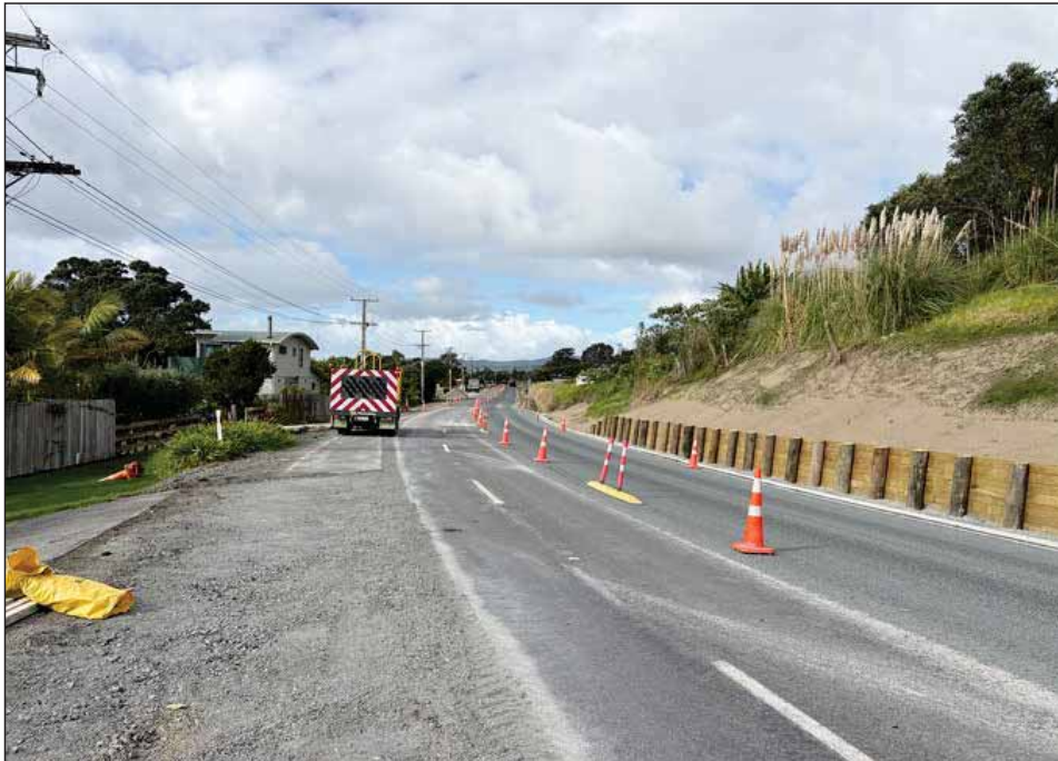
The road realignment is complete
