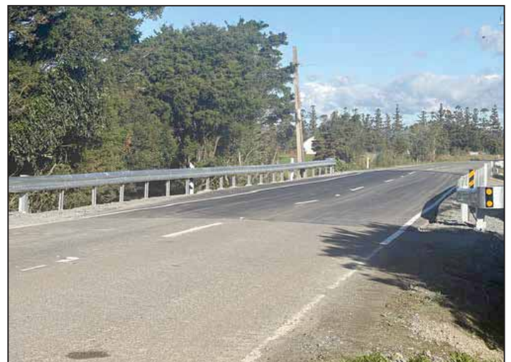
The new Rosyth Rd. Bridge.
